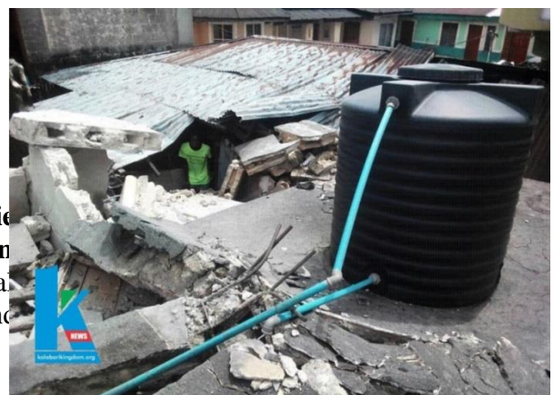
Fig 2.0: Building Collapse in Buguma City
