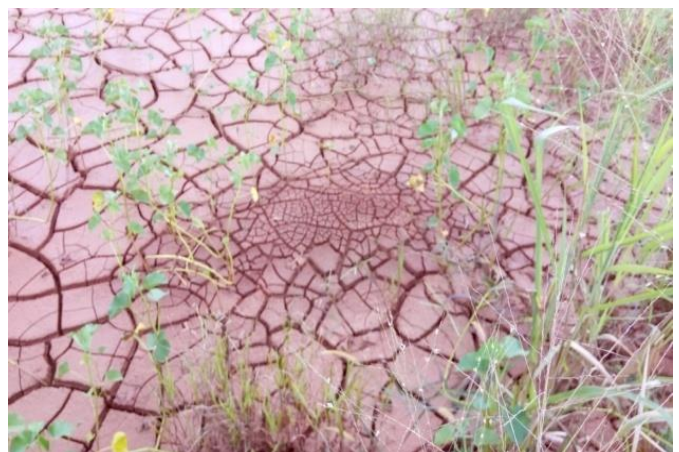
Fig. 1: Mud cracks or desiccation cracks of dried swelling soil.
