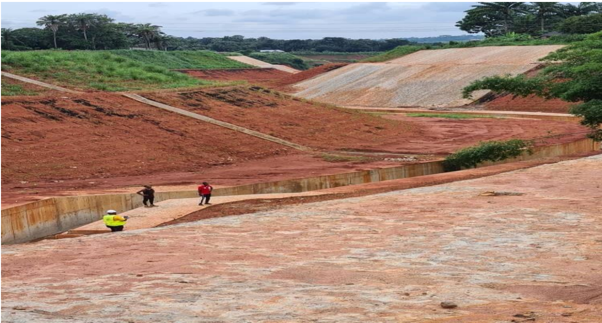
Plate 3.1b: Nnewichi Gully Erosion Site, Nnewichi after intervention.
